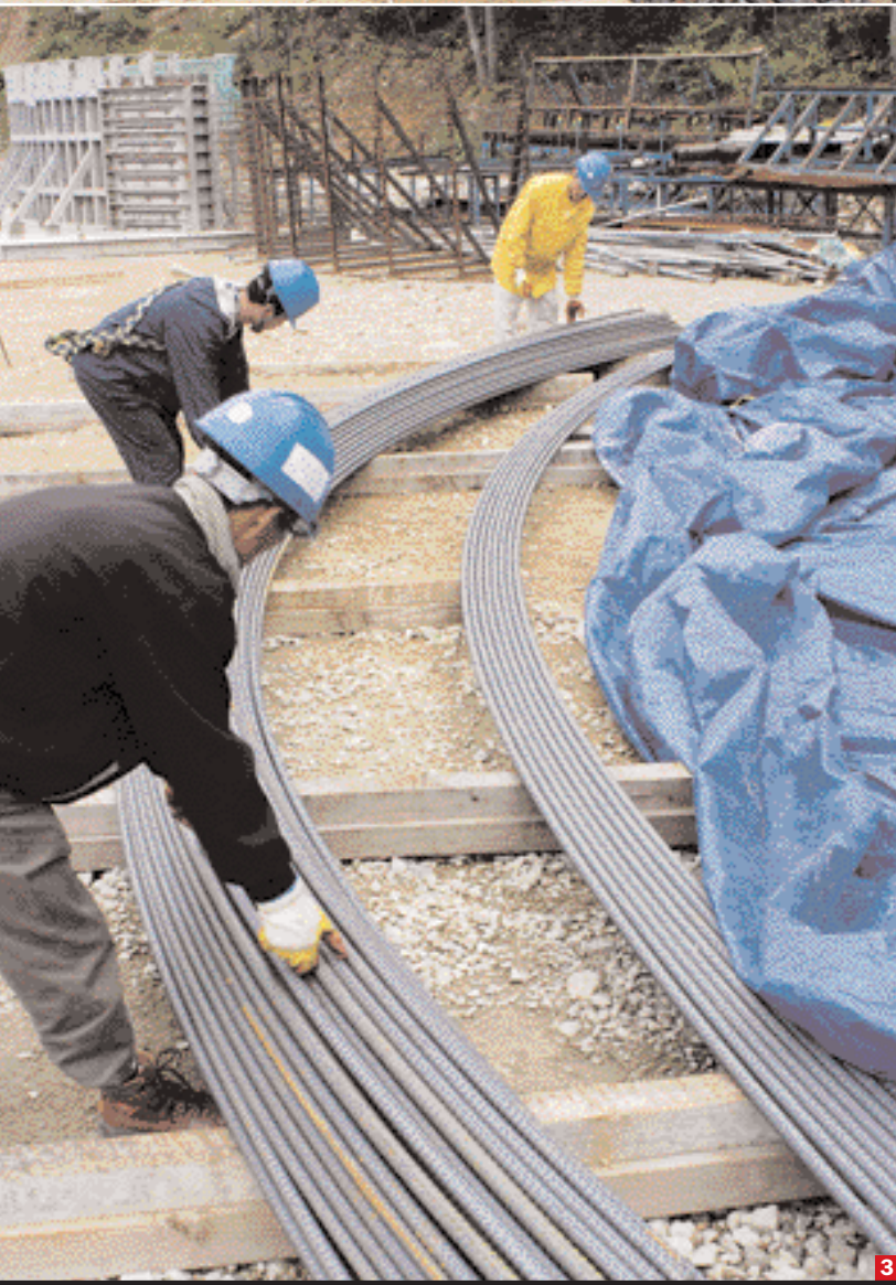
1. The Naeseo 1 double tunnel consists of 256 TechSpan half-sections and is 135 m long. All that remains is to install 15 m of backfill. 2 and 3. Preparation of the reinforcement cages for the TechSpan units . 4. Arch element storage area.
