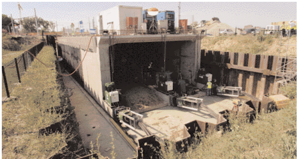
Installation of a railway bridge in Saint-Rémy (Saône-et-Loire) by jack-assisted Autofonçage®.
