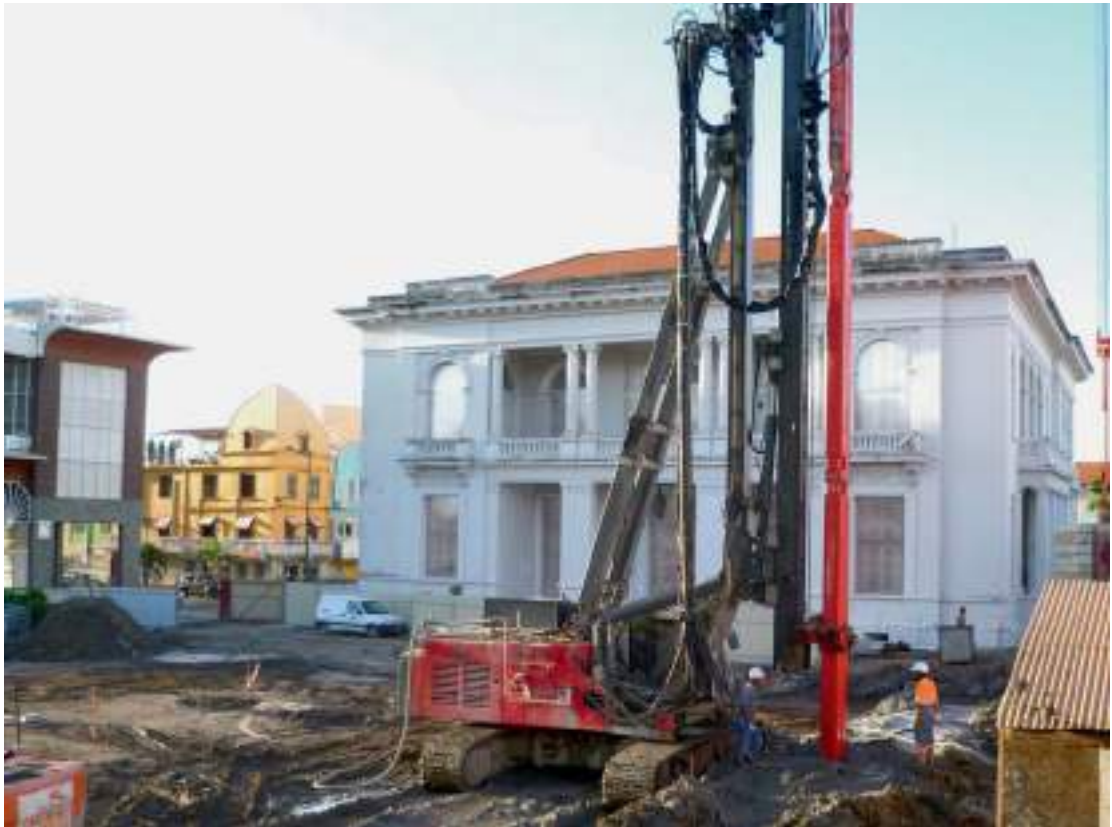
A grid of Geomix® retaining walls will provide earthquake protection for the new buildings.
