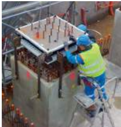
01 - 02 NTI-ABS anti-seismic bearings developed by NTS were used in the RJH and Iter projects.
