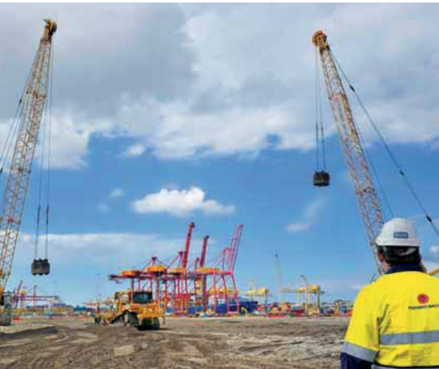
PORT BOTANY , an emblematic Menard Bachy project in Australia.
