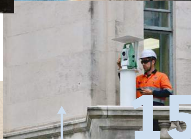
City Rail Link Auckland, New Zealand
