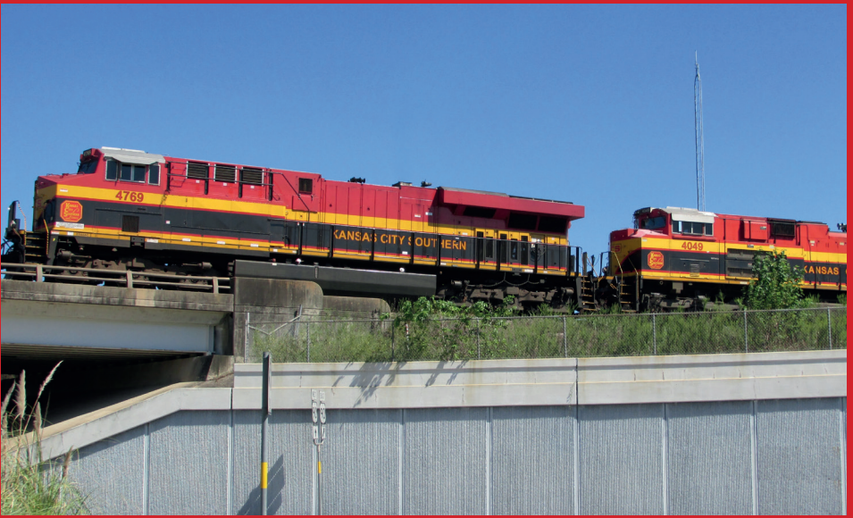
Spur 380 Kansas City Southern Rail Interchange, USA
